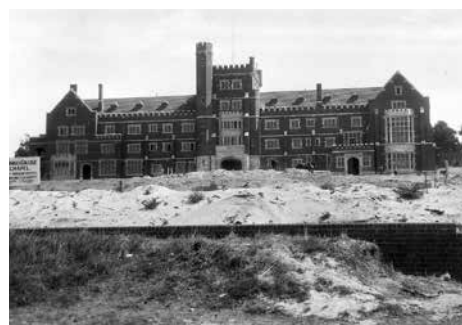
The College under construction
