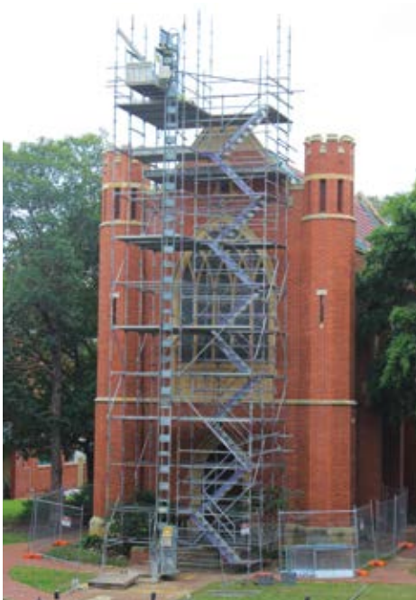
Chapel under repair
